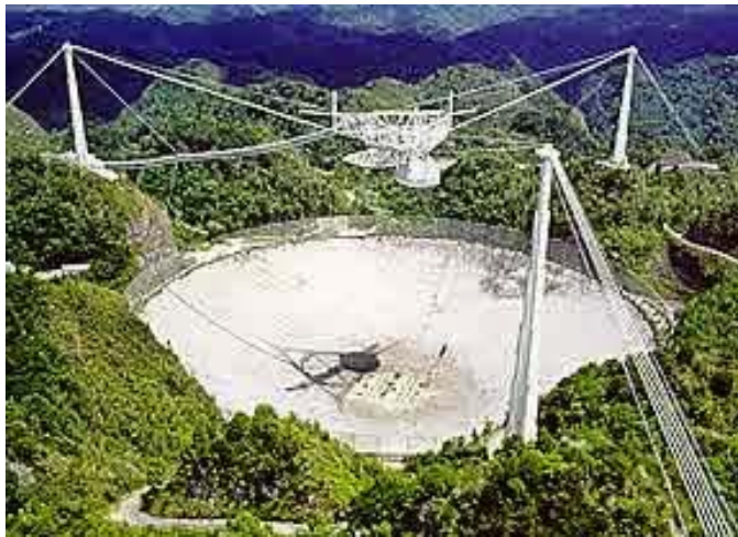
Figure 12-47 Elevation cross section of 305-m diameter fixed spherical reflector suspended in mountain valley at Arecibo, Puerto Rico.
