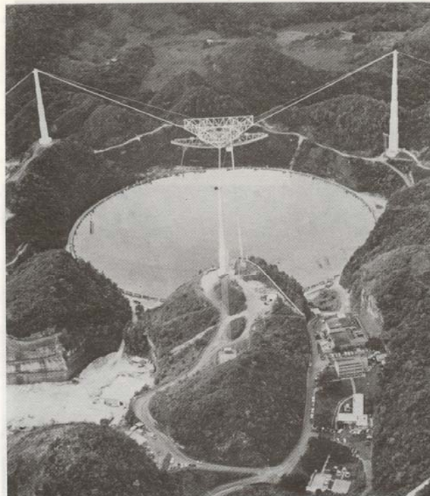
Figure 12-48 Air view of 305-m Arecibo dish. Feed structure is supported by cables from 3 towers. Beam steering by moving the line feed allows observations at angles up to 20^\circ from the zenith. Away from the zenith, only part of the reflector can be used with resulting decrease in aperture efficiency. (Cornell University.)
